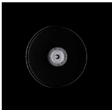
TEY p. 110 EMERGENCY ESCAPE LIGHTING
